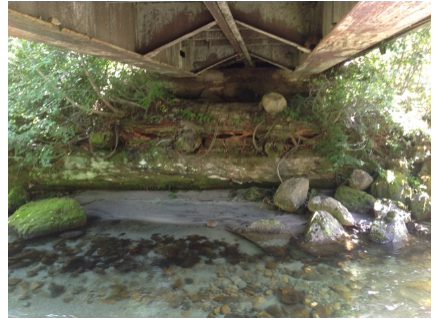
right bank log crib supporting railcar
