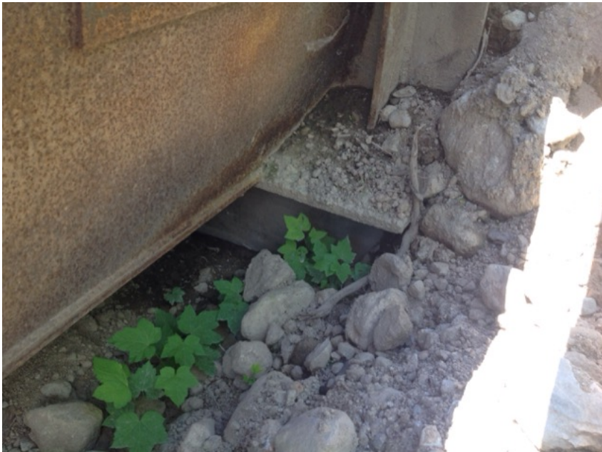
Left Bank Abutment when facing downstream
