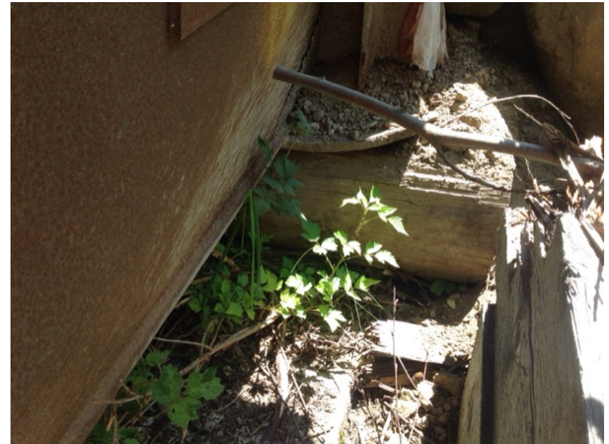
Right Bank Abutment when facing downstream
